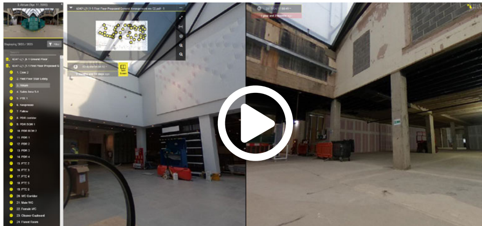
Watch this video to see how Mace Construction uses HoloBuilder to compare documentation captured over time.
