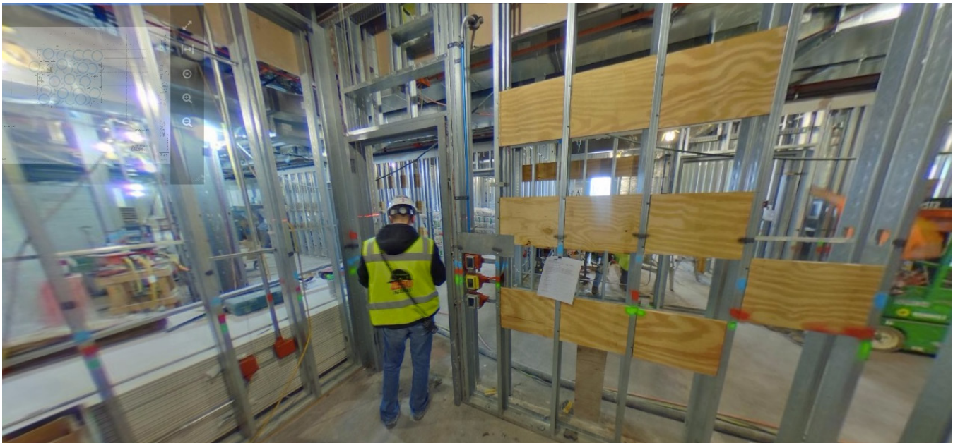
Fig. 1: HoloBuilder view showing a field engineer capturing a 360° photo on-site.
